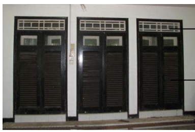
DESIGN OF TIMBER LOUVRES/ GLAZED DOOR AND TIMBER LATTICE TRANSOM AT 1 ST STOREY
