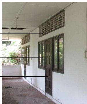
INNER FAÇADE OF 2 ND STOREY BALCONY
