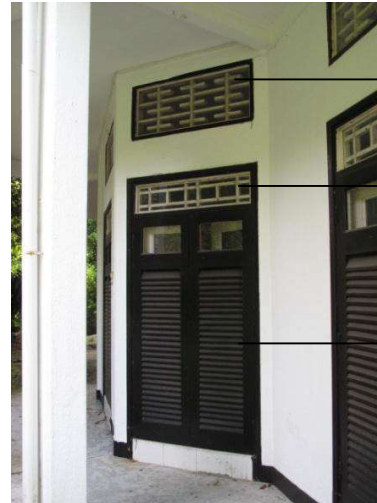
DESIGN OF TIMBER LOUVRES/ GLAZED DOOR WITH TIMBER LATTICE TRANSOMS AND TIMBER LATTICE VENTS
