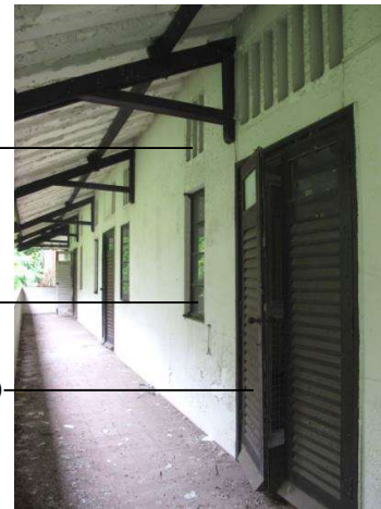
INNER FAÇADE OF 2ND STOREY BALCONY
