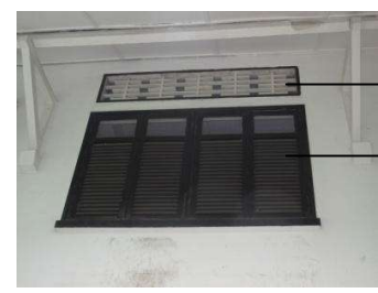
DESIGN OF TIMBER LOUVRES/ GLAZED WINDOW AND TIMBER LATTICE VENTS AT 2 ND STOREY
