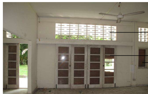
1 ST STOREY (view from inside)
