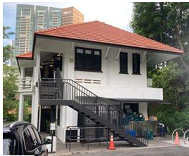
✓ Acceptable exhaust duct (visually neat/blend well with the bungalow)
