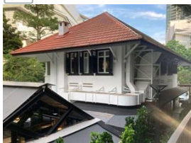
✗ Non-acceptable exhaust duct (visually cluttered with inconsistent shape and multiple braces, blackish duct that requires regular maintenance and repainting)
