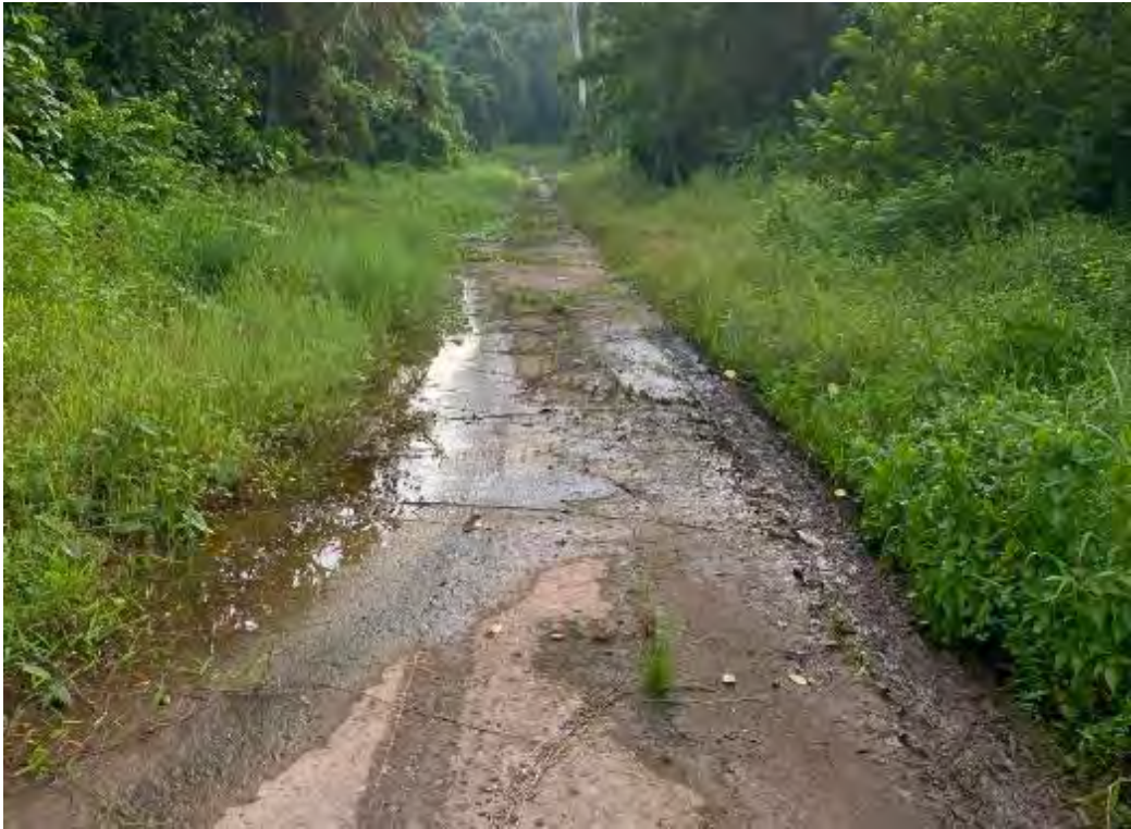
Figure 8.19 Example of water seepage from north of A14 flowing towards A14.
